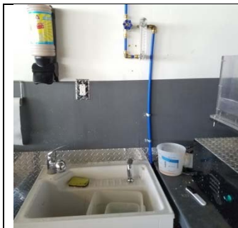
Example of a Flow Regulator and Shower Head Rinse Apparatus
